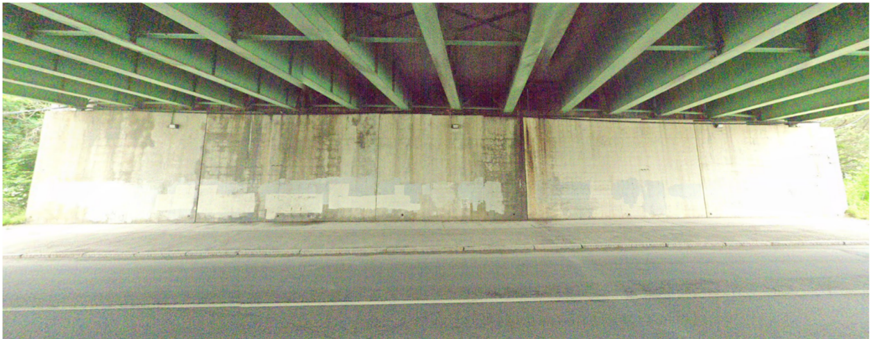
Photograph 1 – Abutment No. 1 (west side of existing bridge) supported on steel HP 14x89 piles.
